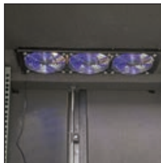
3 x Super-Silent fans in roof area
