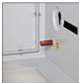
Central grounding bolt
