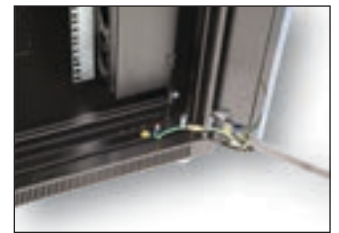
Doors and side walls are earthed
